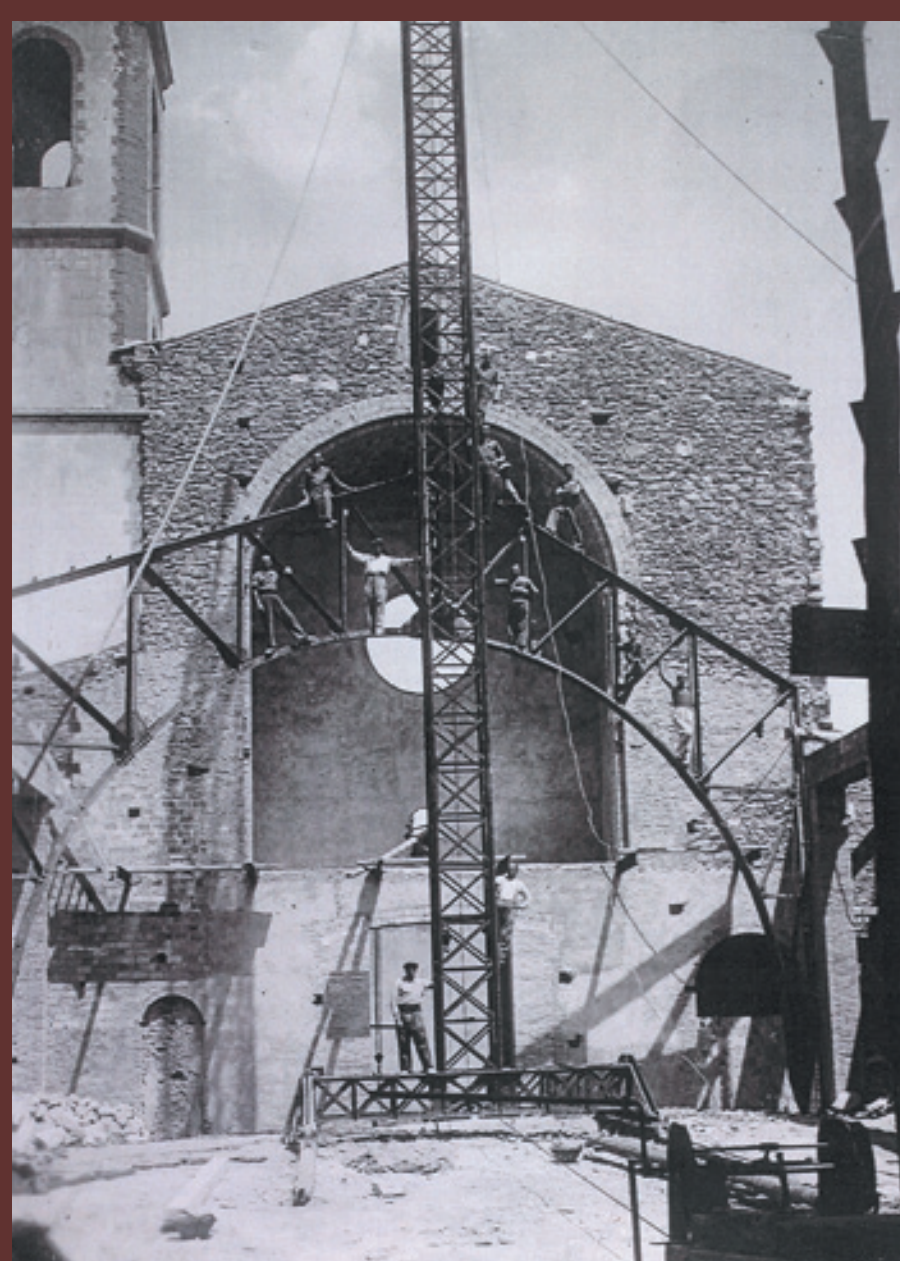
Reconstruction work on the church. Construction workers posing on an iron frame [Unknown author / Tona Municipal Archive. L'Abans Collection. Ramon Batllés Archive Collection]
